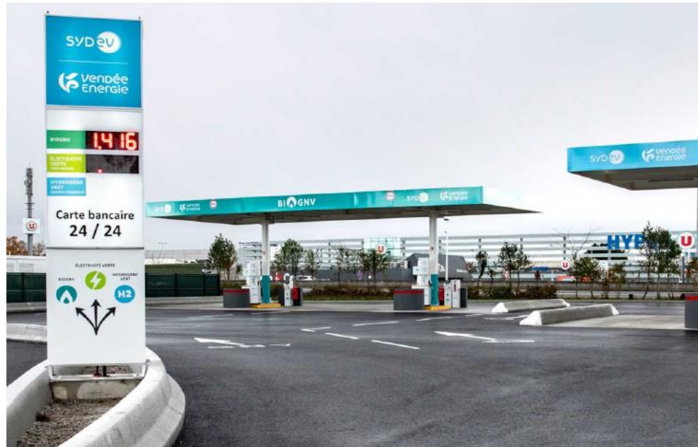
Station multi-énergies, La Roche-sur-Yon (85)
